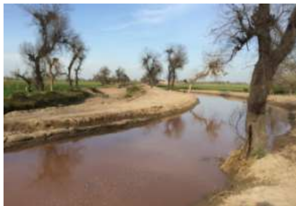
Photograph No. 5: View of the constructed diversion channel through temporary land occupation at ICB-05 (RD 59+200) in village 18/11-L..
