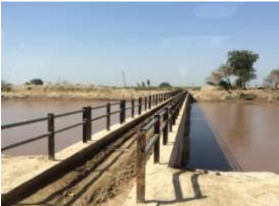
Photograph No. 7: View of the newly constructed foot bridge at LBDC main canal.
