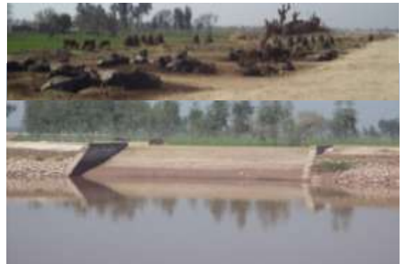
Photograph No. 10: A view of newly constructed Cattle ghat (bafloes Ballow) on the LBDC main canal.
