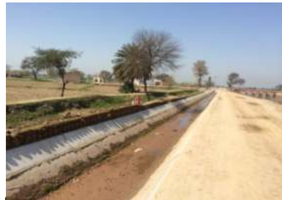
Photograph No. 6: View of the newly lined distributary under ICB-04.
